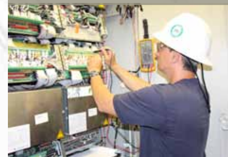
Guthrie works on equipment at Silver Creek.
